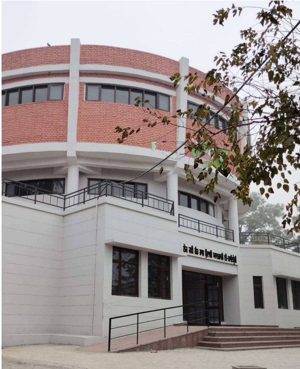
NEW LIBRARY OUTSIDE VIEW
